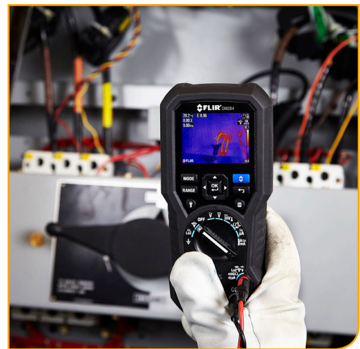
Thermal scan of an electrical panel
